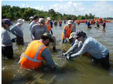
Jacobs was commissioned by The Nature Conservancy (TNC) to undertake analytical and design services for the Arlington Cove Living Shoreline Project. The project involved the design of offshore reefs comprised of precast concrete oyster reef units, for coastal erosion protection along 2.5 km of shoreline. The project aimed to deliver habitat enhancement, provide shoreline protection, and promote marsh accretion and re-growth by reducing wave energy in the lee of the new reef breakwaters.
